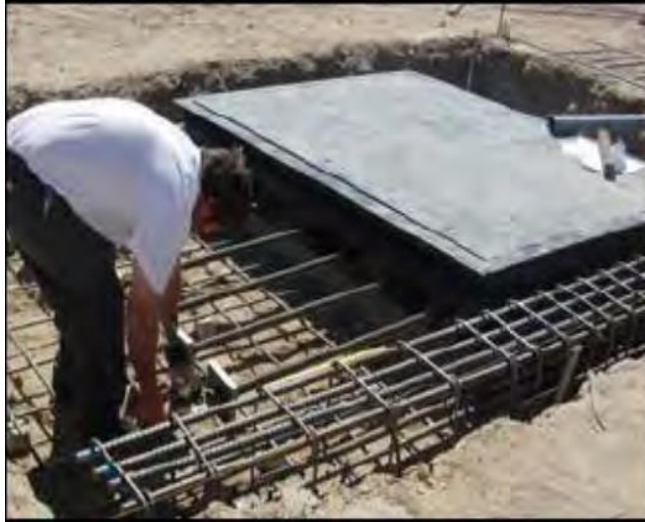
Picture 6 - Tie down Side Beam Reinforcement
