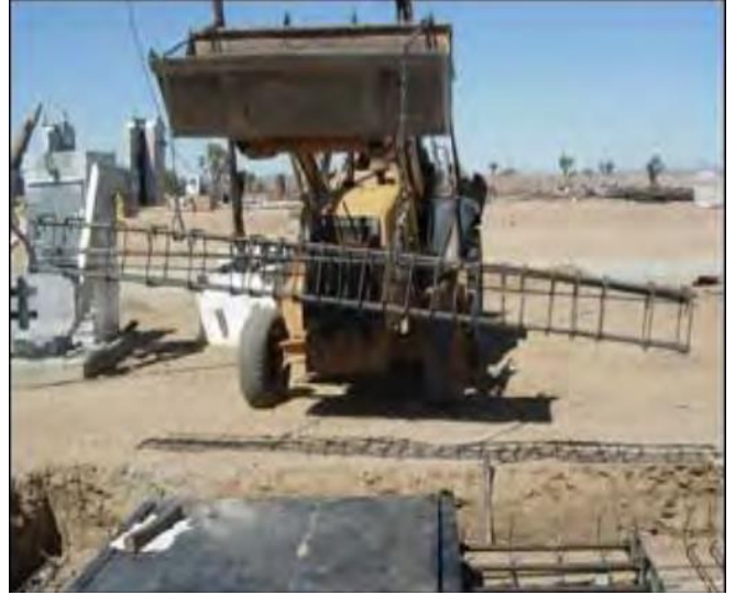
Picture 5 - Pre-Assembled Side Beam
