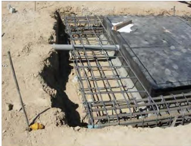
Picture 7 - Top Layer Rebar
