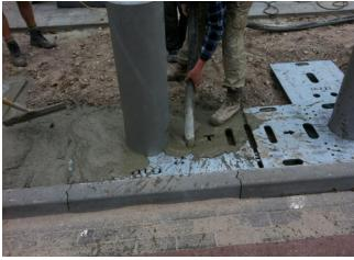
The concrete should be poured flush with top plates and biscuits and clear of excess concrete.
