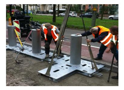
Lift the bollard into position. Ensure it is level and bollard is vertical. This will make it easier to join the next bollard.
